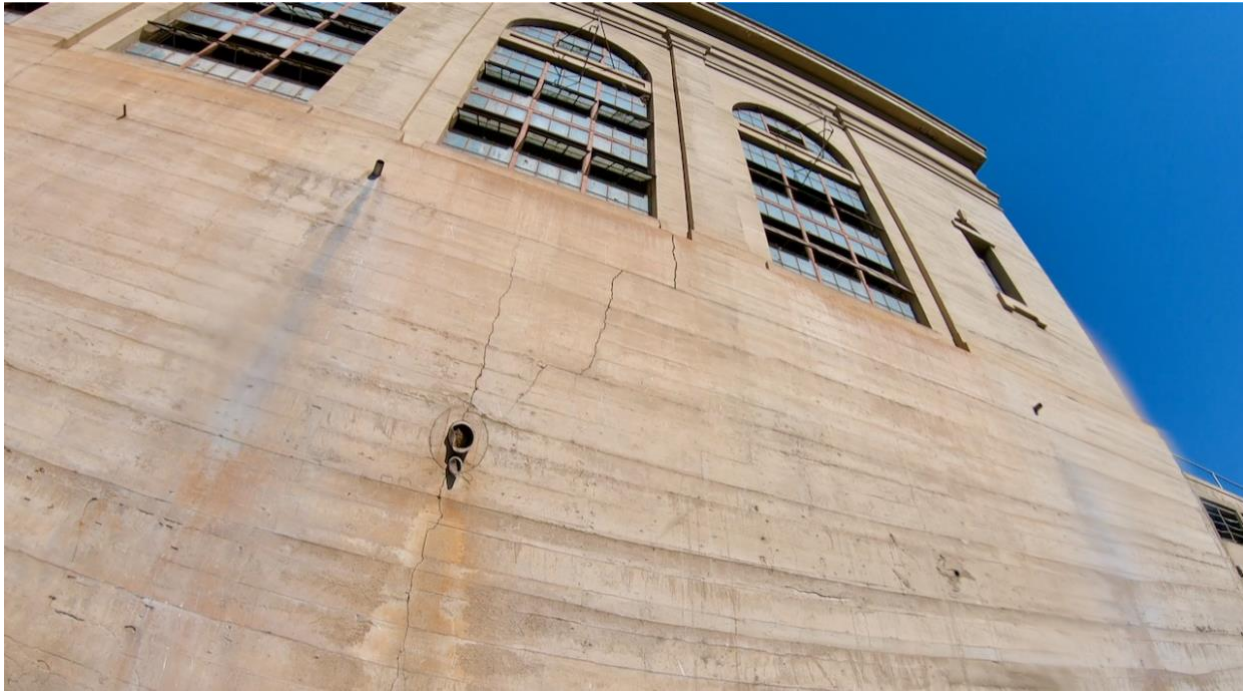
Figure 60: The Powerhouse and the Security Fence
