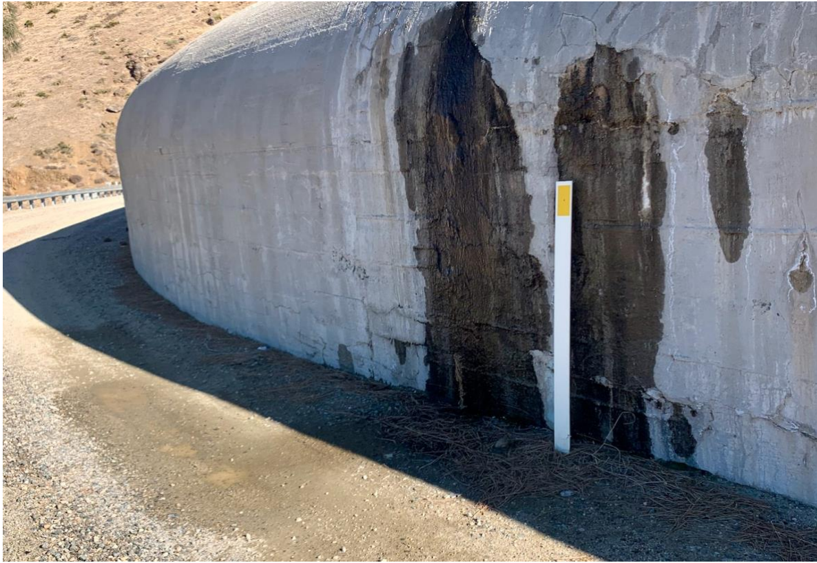
Figure 59: KR3 Conveyance, December 02, 2021
