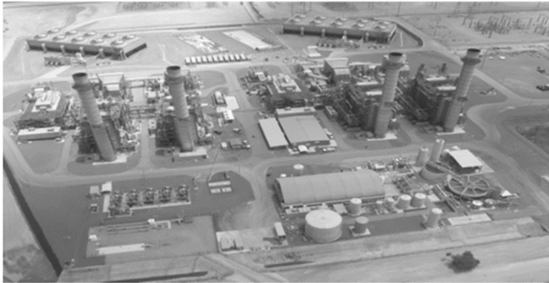
Figure III-4 Mountainview Generating Station
