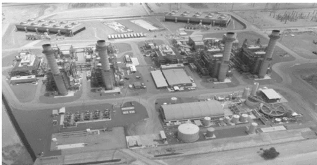
Figure III-13 Mountainview Generating Station
